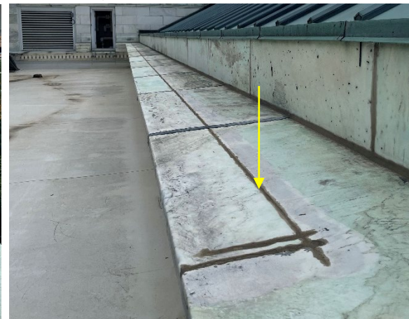
Horizontal joints on cornice stones
