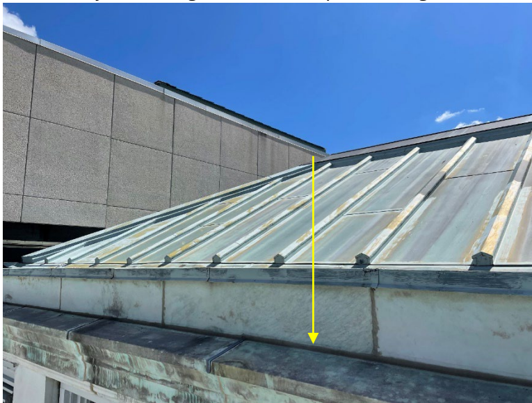
Horizontal joints along the cornice capstone ledges
