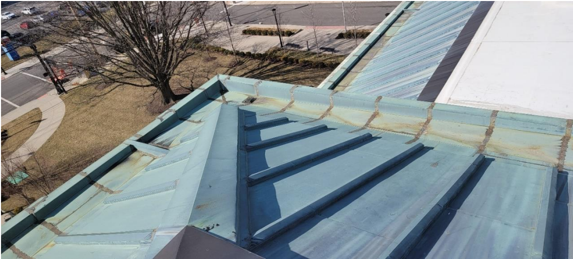
Integral Box Gutter center portion northwest corner
