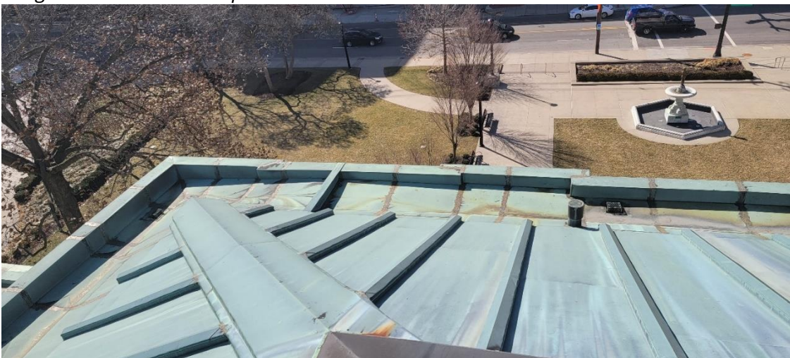
Integral Box Gutter center portion southwest corner
