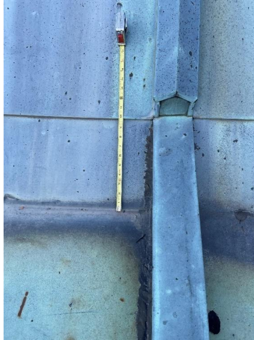
Gutter Slope Height
