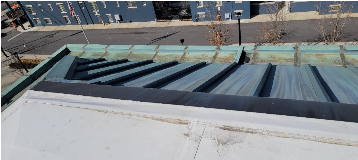
Integral Box Gutter north wing north face
