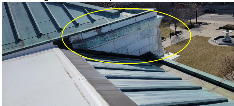
North facing vertical marble panels
