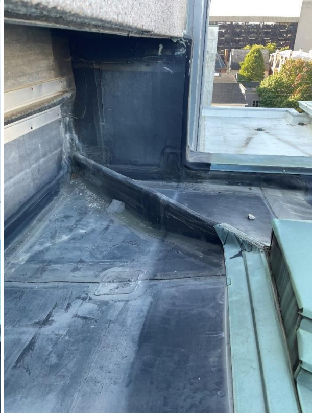
East wall southeast corner looking south
