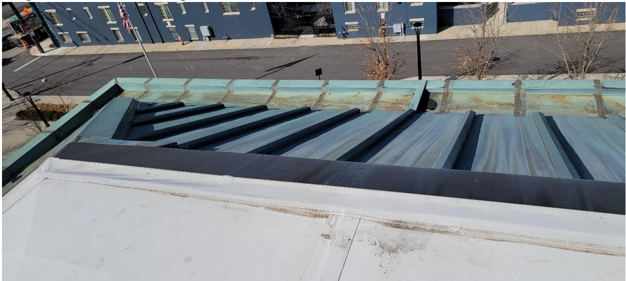
Integral Box Gutter north wing north face
