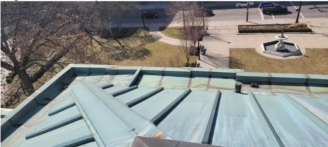
Integral Box Gutter center portion southwest corner
