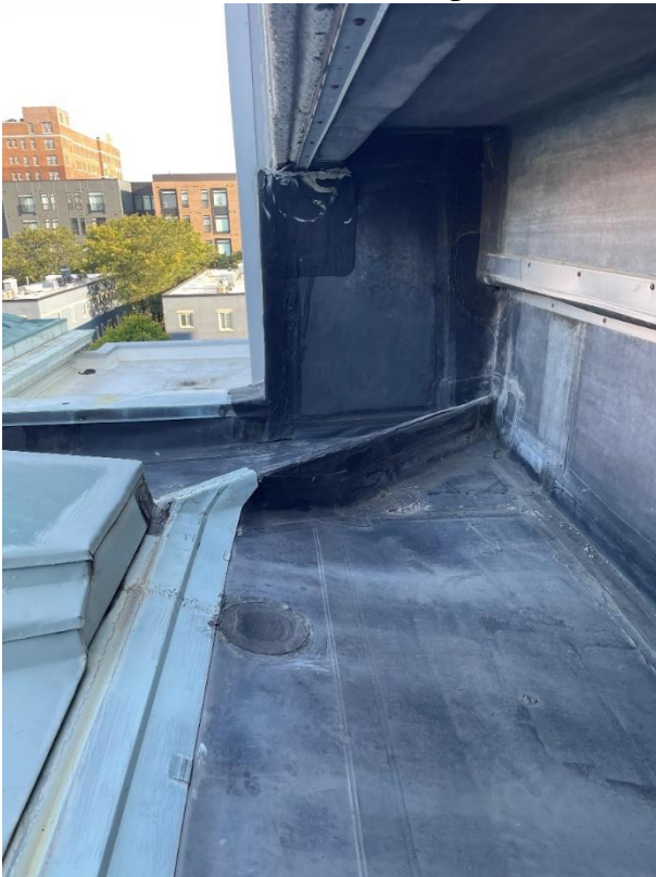
East wall northeast corner looking north
