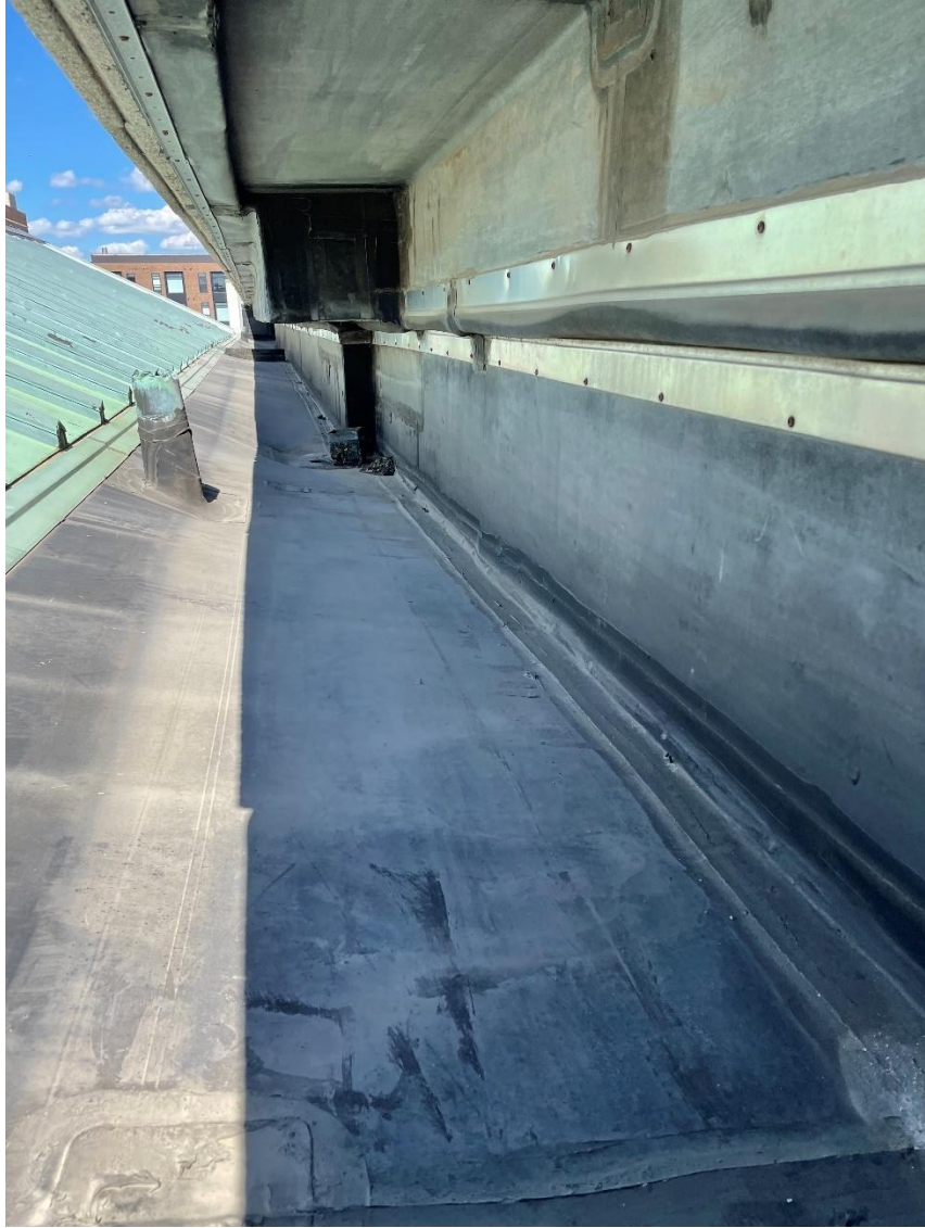
East wall looking north
