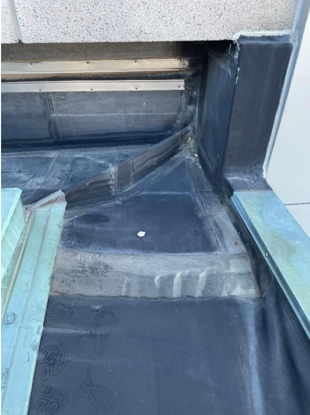
East Wall southeast corner looking east
